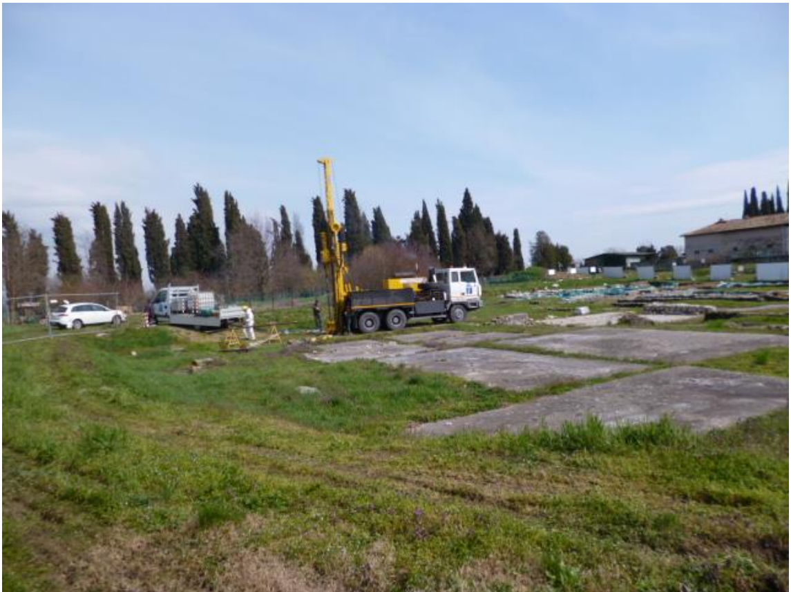
Sonda Gelma 2, sondaggio S1 – SRV srl – 2013
